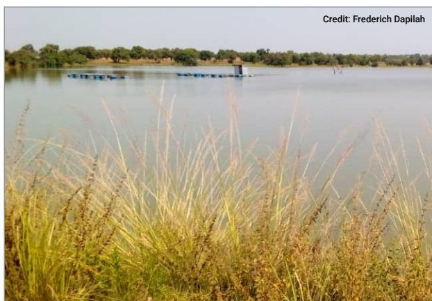
Photo 5.5. Irrigation Dam at Datuko, Upper East Region
